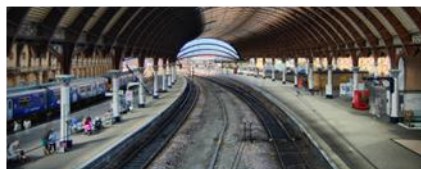
A LEADING RAIL HUB IN EVERY WAY
